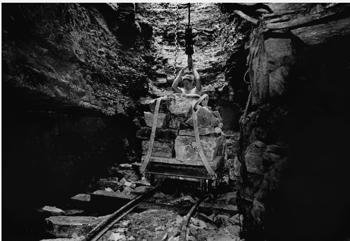
At the foot of the vertical shaft the crane hook is about to be attached to the slings which are attached at the corners of the flatbed cart. 1982.
